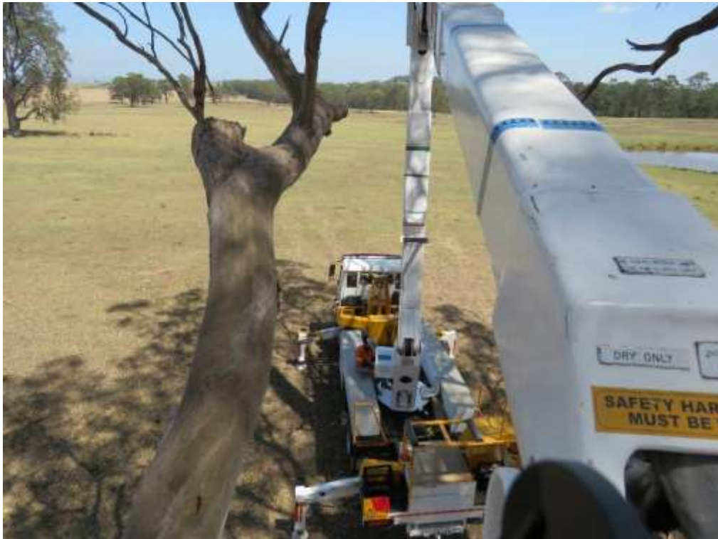
Plate 2. View from cherry picker at HBT 8 showing spouts that are shown in Plate 4.
